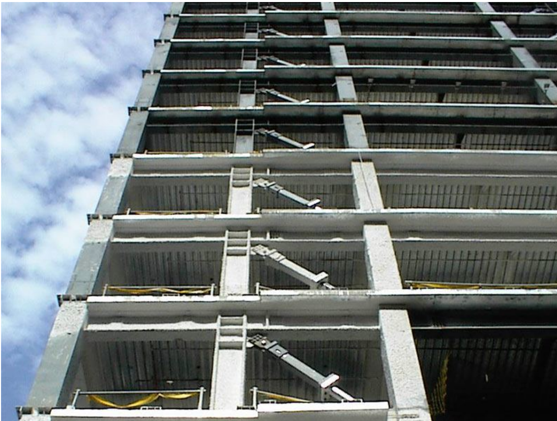
Figure 1: Buddhist HQ (Taipei, Taiwan) equipped with viscous dampers
